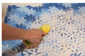
8. Apply the grout to the tile sheet surface
