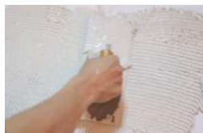
4. Apply the adhesives to the substrates
