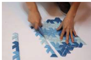
6. Cut off the excess and fit the mosaic edge
