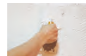
4. Apply the adhesives to the substrates
