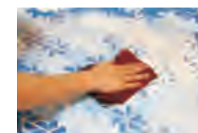
9. Use a soft towel to remove excess adhesive on the surface
