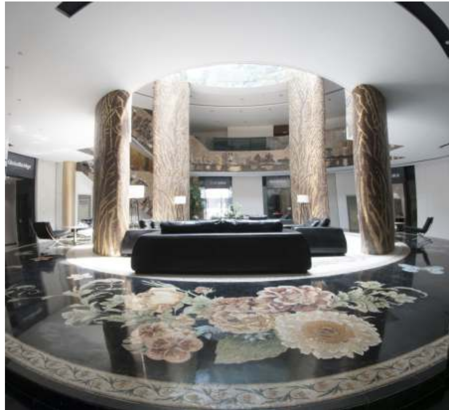
Annular stone mosaic flower wall puzzle. The entire circular floor uses stone mosaic with hand-cutting, water-jet cutting, self-leveling cement. It is a typical case of various materials and multiple processes production and installation techniques application.
